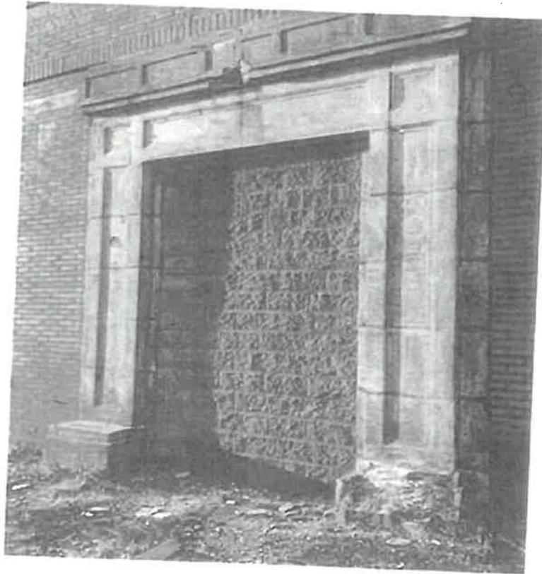
EXHIBIT "C" Doorway located along W Fifth Street
