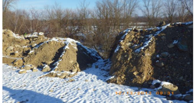
Runoff from the street/spoil area is directly tributary to Rock Fork.
