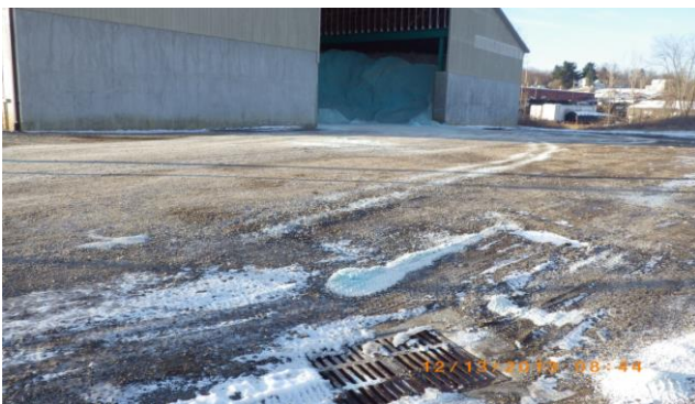
Stormwater inlet where runoff from loading activities flows into.
