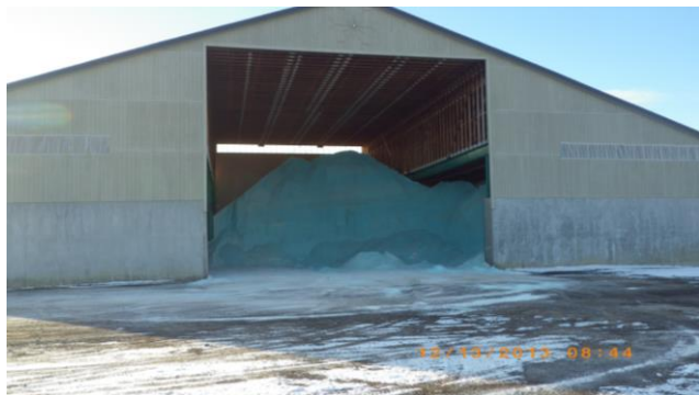
Salt barn entrance located along the northwest perimeter of the site.
