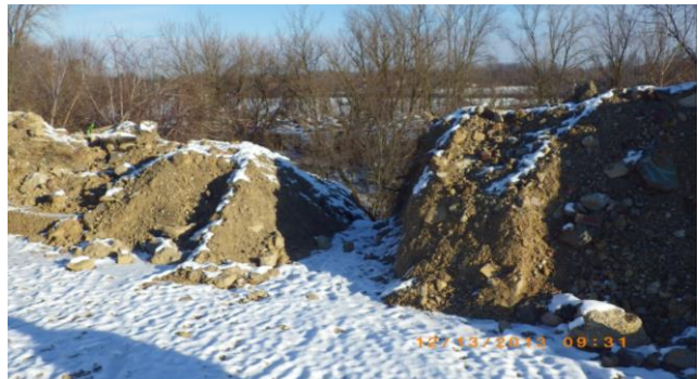
Runoff from the street/spoil area is directly tributary to Rock Fork.
