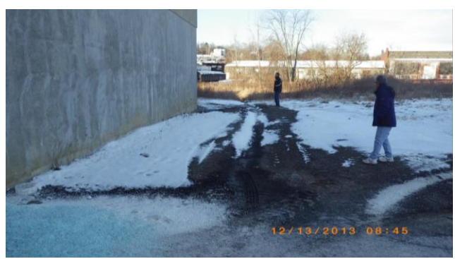
Ditch outside of Salt barn leading to the retention area.
