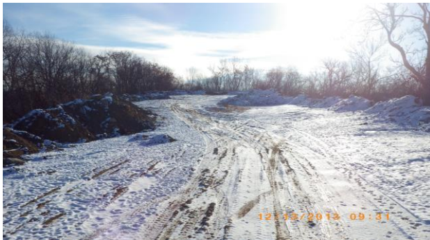
Street/Sewer spoil area.
